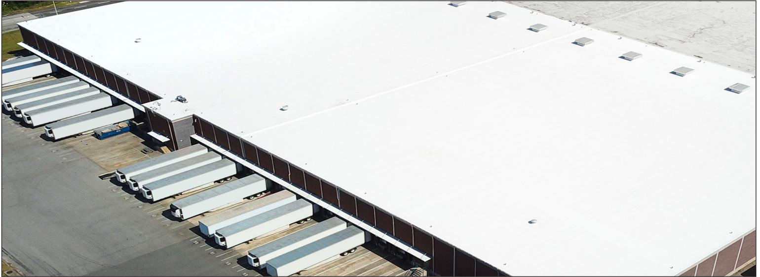
This industrial warehouse facility is a fully leased 540,000 sq. ft. building. The final phase of re-roofing was scheduled over difficult-to-fasten-to decks (a combination of lightweight insulated concrete and tectum). With a desire to control costs while minimizing tenant disruptions, the final and largest re-roof phase was designed using a combination of vented roof and tear off configurations.
